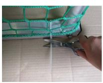
c) Fix net at the bottom of net hoops with 3 cable clips. Cut projecting parts.
