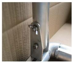
h) Press net hoop to the outside. Stick from the top hexagon screw DIN 933, M 8 x 60 through the 2nd borehole of the upper hinge and the hoop. Then add washer DIN 125, Ø 8.4 mm at the hinge lower side and screw wing nut DIN 315, M 8.
