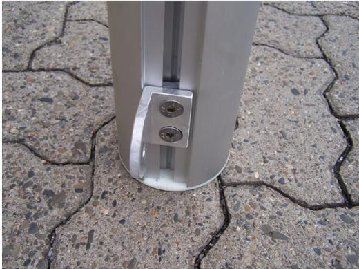
3. Fix uprights in ground sockets, adjust hinge part and tighten all screws.
