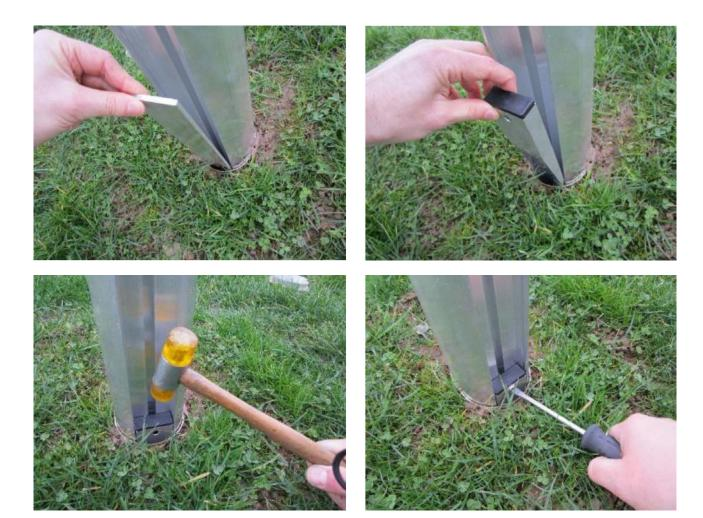
b) Set mounted goal with fixed ground sockets in the foundations (80x80x100cm). To enable a drain off of possible water we recommend to stick a tube each below the boreholes of the ground sockets. After careful adjustment of the goal to the side and specified height by crossed bars pour concrete into the foundation ditches.
