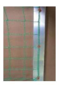
b) Dismantling of the net is also done by rotation of the net holders through 90 degrees. Use again a screw driver if necessary.
