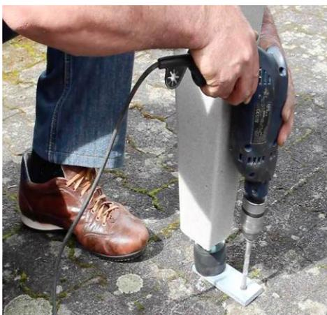
Lift one side with two persons using one of the delivered squared timbers. Screw the rubber buffers (with the pre-assembled metal straps for floor attachment) into the substructure. Adjust the height. Fix the substructure to the ground using wood screws 8x60 with the dowels.
